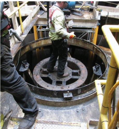
Telescoping supports and scaffolding stabilized the bridge and reaction well during installation.
